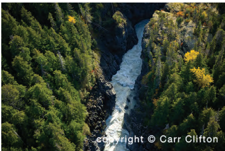
Iskut Canyon on the Iskut River. Water from the Iskut River will be diverted to produce hydroelectric power. Photo courtesy of Carr Clifton.
