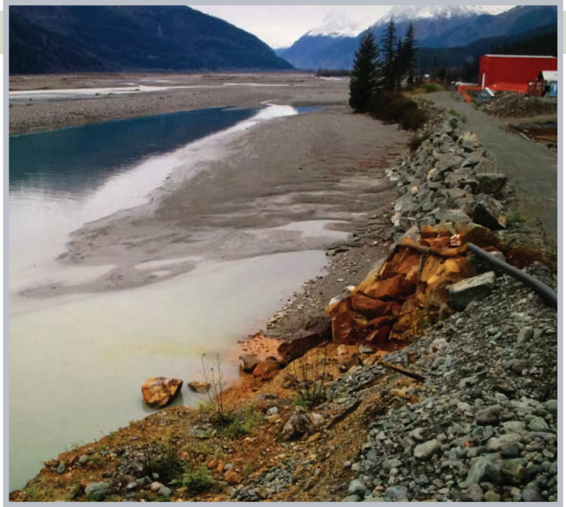
Picture from October 2015 inspection showing acid mine drainage piped directly into the Tulsequah River.
